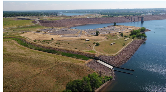
North Boat Ramp following construction that was completed in June 2018.
