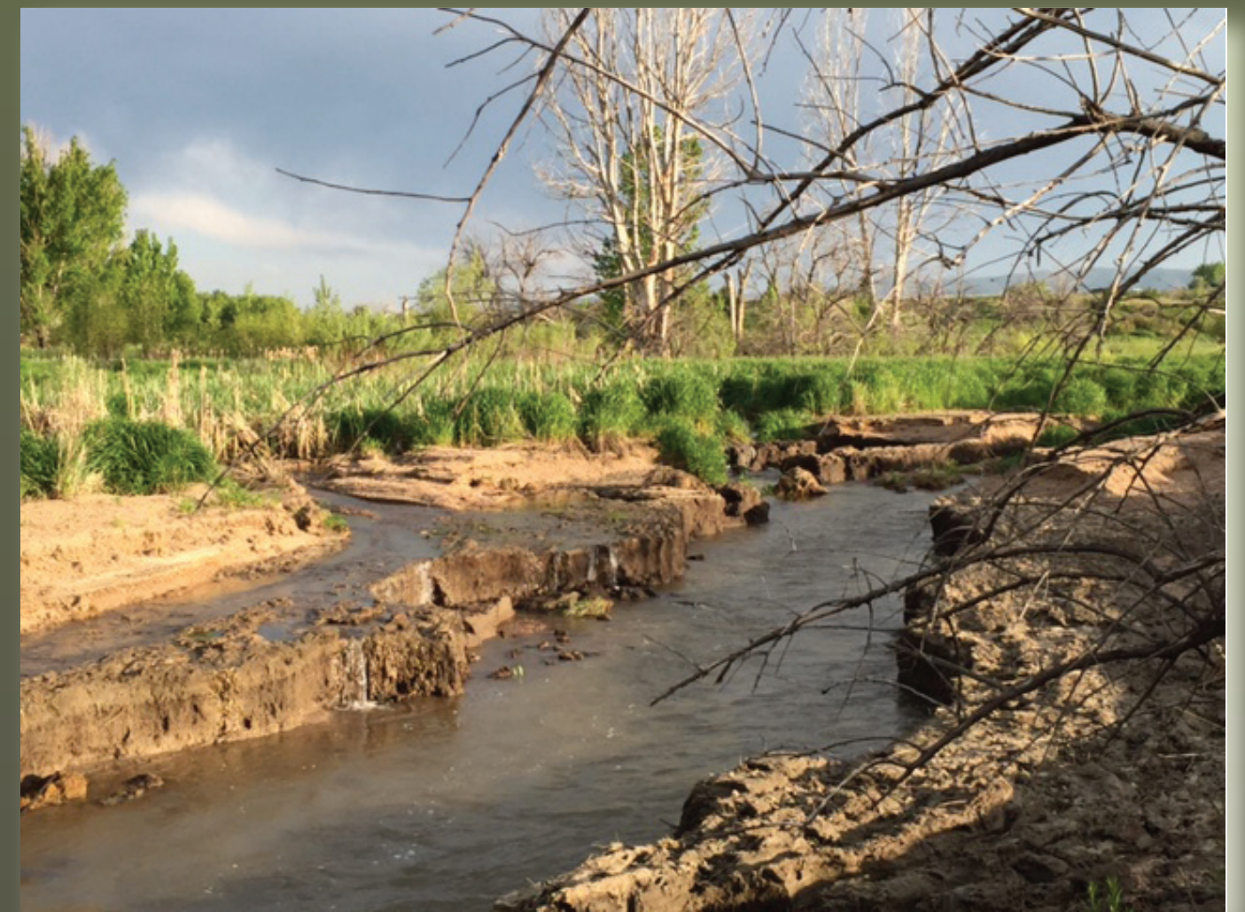
Headcutting along Plum creek
