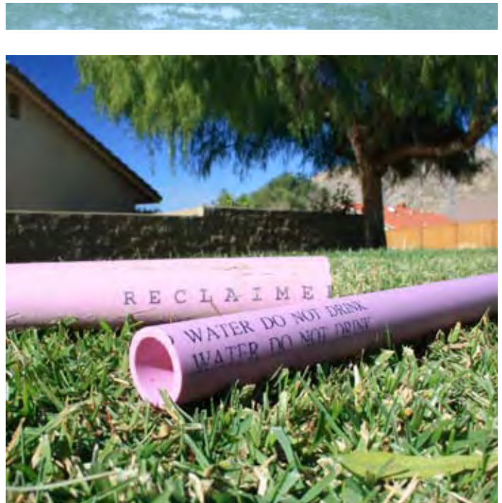
Recycled water projects use "purple pipe" to convey supply from the treatment plant to the point of use.
