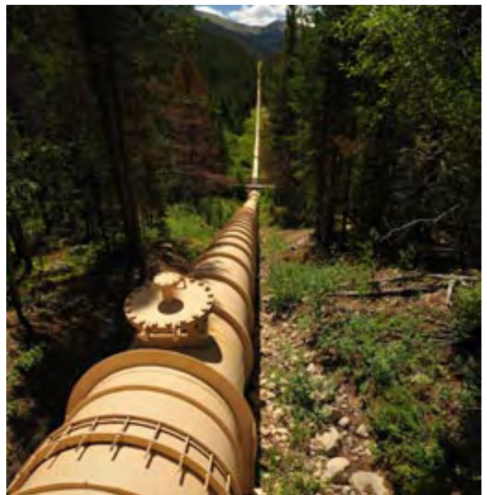
The Moffat Pipeline, part of Denver Water’s Gross Reservoir Enlargement project. Photo: Mark Conlin.
