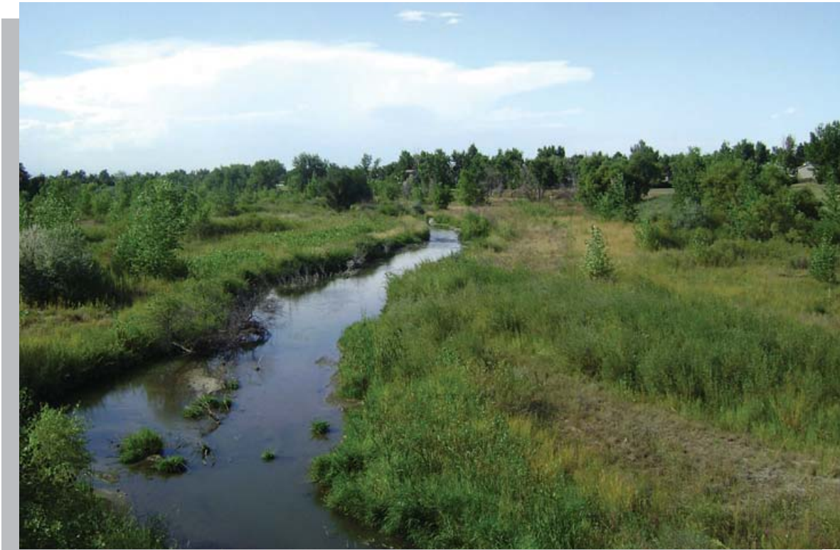
Figure 6 - Cherry Creek at Apache Plume Outfall. Looking downstream at expanded Preble's habitat behind low sheet pile cutoff wall. Cutoff wall is visible at about the middle of the photo, just before the stream bends out of sight.
