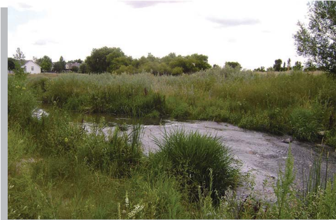
Figure 5 - Cherry Creek at Stroh Ranch stream restoration project. Looking upstream at small riffle structure. Wetlands have expanded upstream of the structure.
