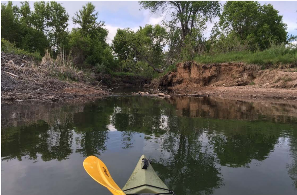
Photo 10. Erosion at Spillway on North End of Titan Lake
