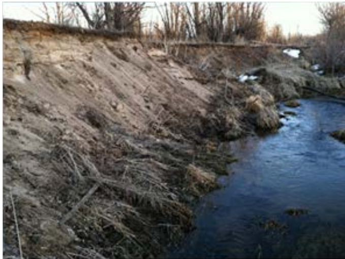
Photo 3. Degradation in the middle channel of Plum Creek had lowered the invert and adjacent water table by approximately 10-feet.
