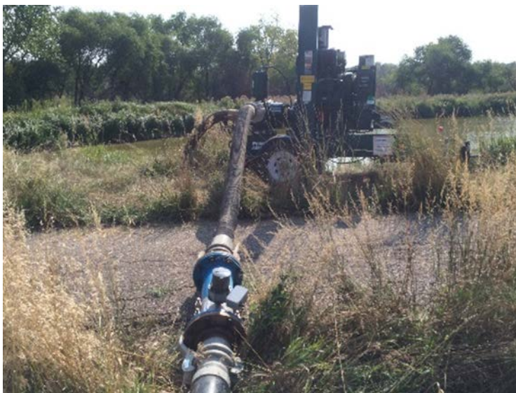
Photo 5. The 6-inch pump used for the field testing provided a flowrate of approximately 1300 gallons per minute (GPM) for evaluating pond drawdown and infiltration capacity.
