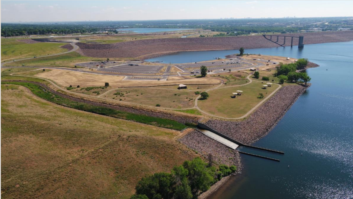
North Boat Ramp following construction that was completed in June 2018.
