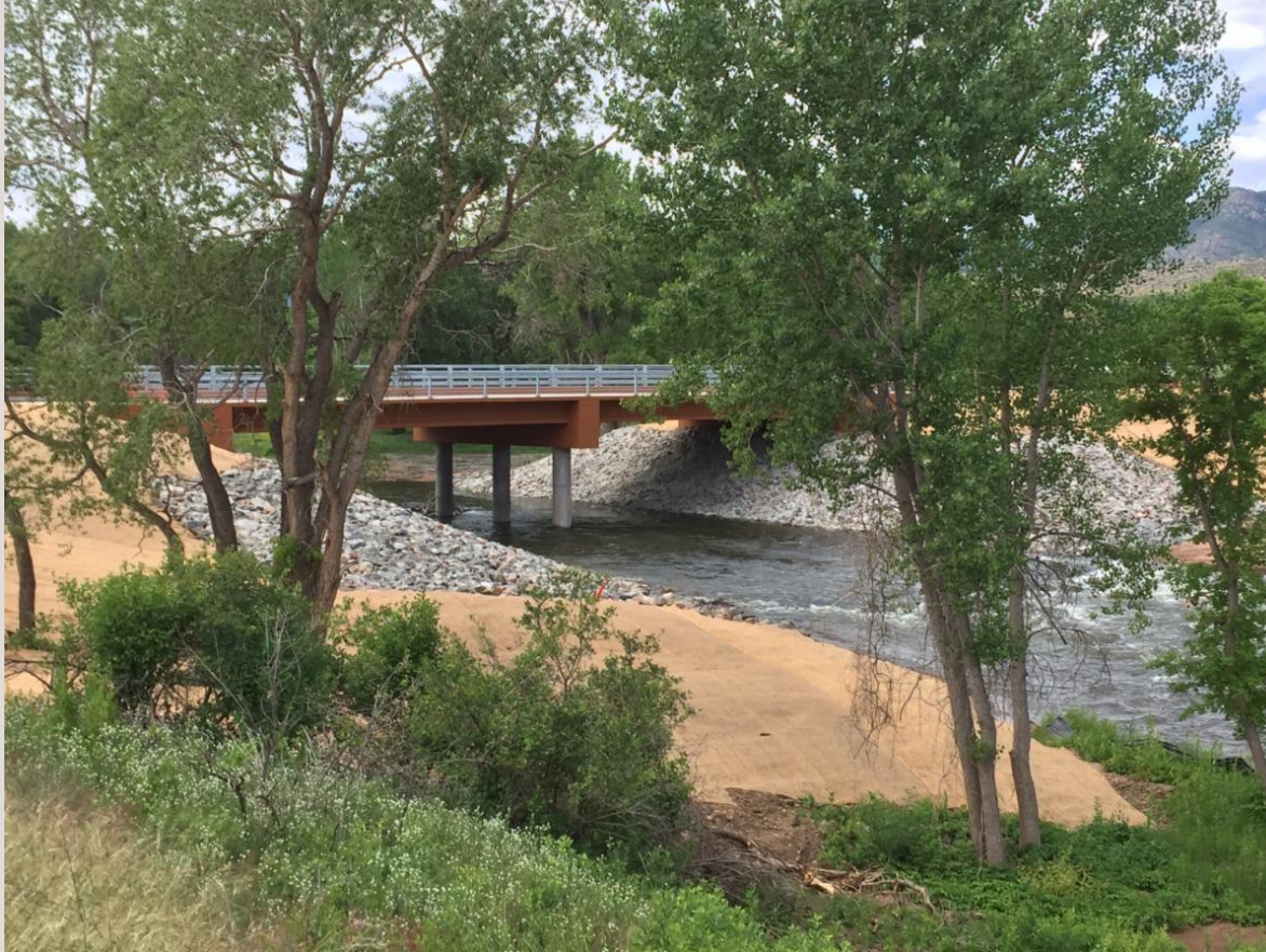
South Platte River Bridge following modifications to accommodate the new reservoir elevation of 5,444 feet.
