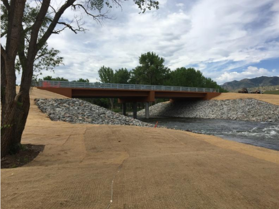
New bridge that spans the South Platte River allows for the reopening of the Perimeter Road on July 3, 2019.
