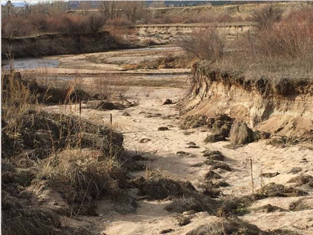
Widespread erosion was evident on Plum Creek throughout the Chatfield State Park reach prior to the implementation of this project.
