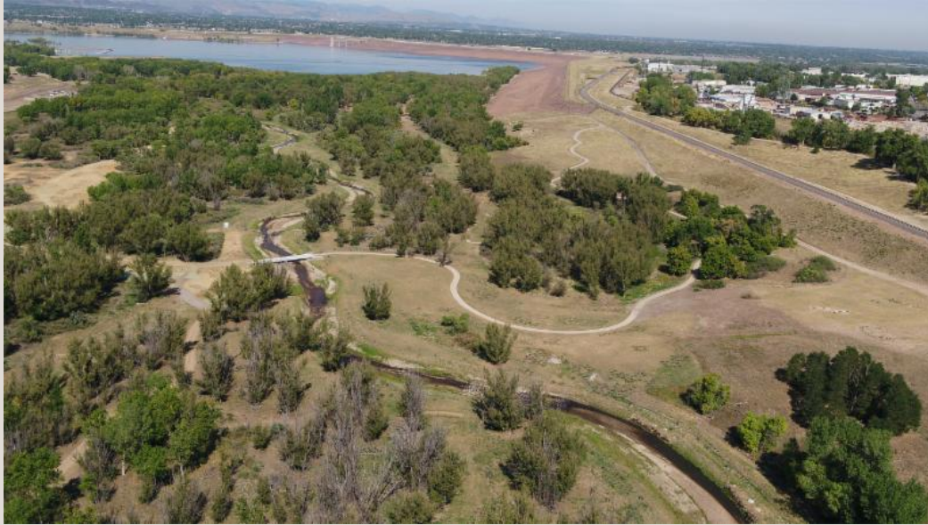
Downstream view of the new Plum Creek Trail connection that provides for the first time a new loop around Chatfield Reservoir.
