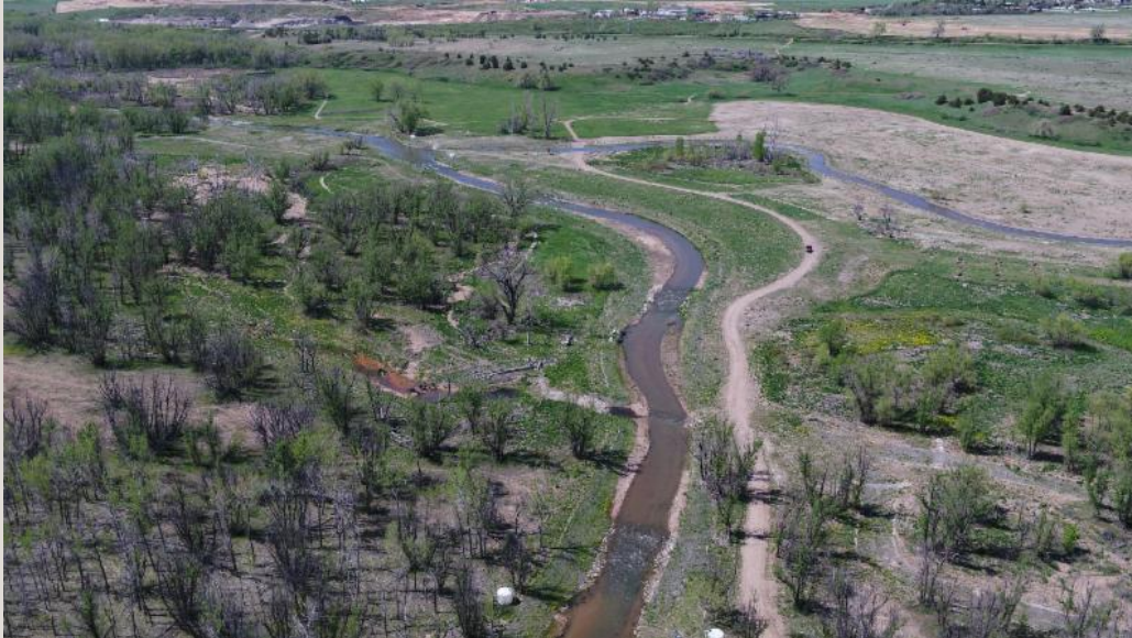
Aerial view of the completed Plum Creek main channel work showing several riffle-drop rock structures installed to eliminate erosion and channel degradation.
