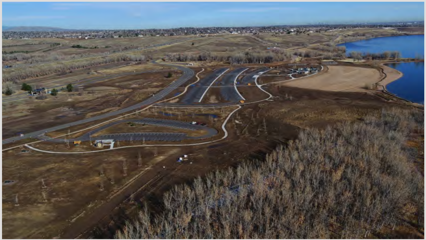
Newly constructed Jamison Day Use Area and Swim Beach, which will open Memorial Day Weekend 2019, from the air. (NOTE: Jamison Day Use Area opened on October 1, 2018.)
