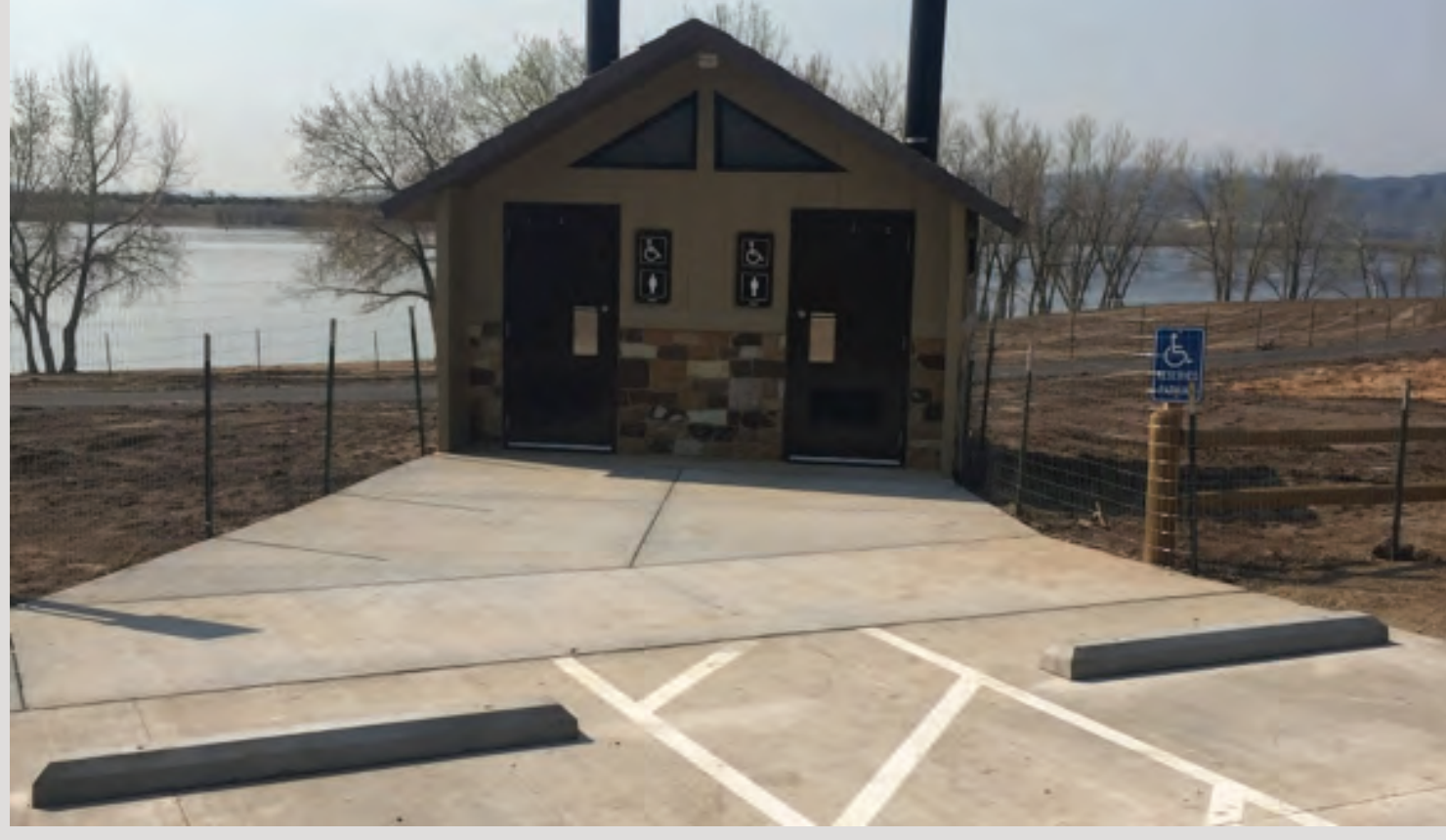
New Massey Draw Day Use Area is now open to the public.
