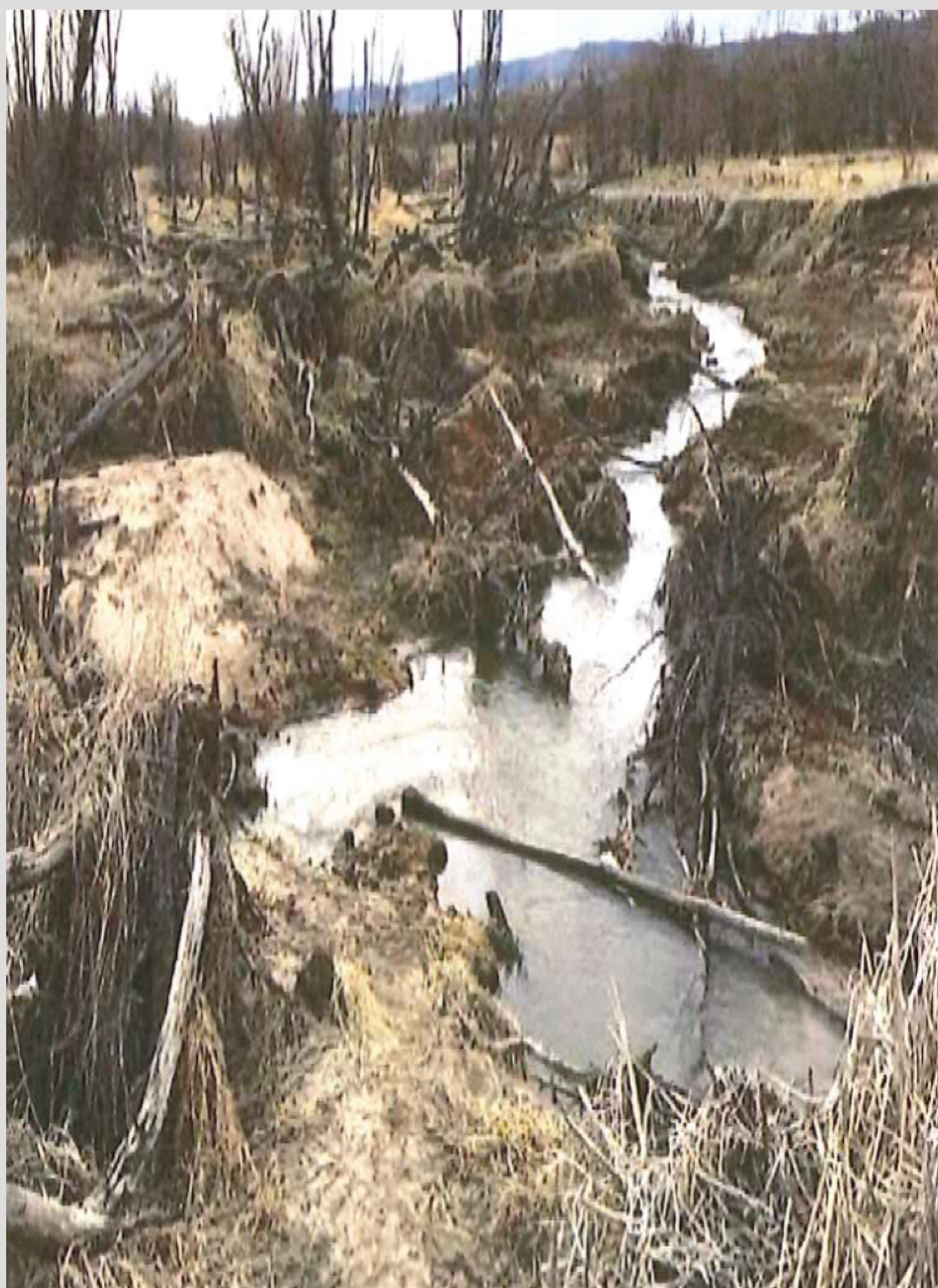
The Plum Creek corridor, from the new higher water level of the reservoir, upstream approximately 7,000 feet, will be stabilized by raising the multiple stream bed sections and constructing riffle-pool rock structures to control longitudinal grade and planting of riparian and wetland vegetation to control erosion and provide habitat.
